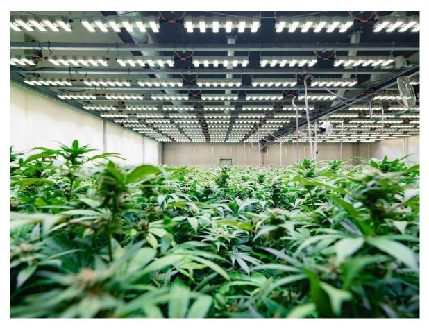
Combined with red LEDs for horticulture lighting, white LEDs provide the right spectrum for the growth of various plants.
