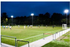
The new high-efficiency pitch lighting consists of 12 Siteco Floodlight 20 Maxi LED units with two different light distributions.
