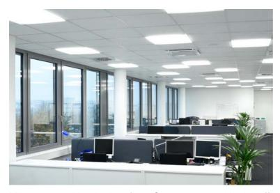
Mira recessed luminaires from Siteco are used in the offices, controllable in light colour and light intensity via Tunable White functionality.
